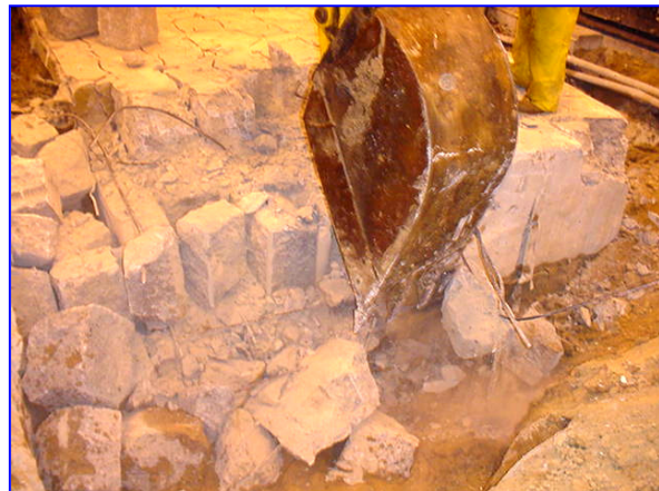
Digging fractured foundation with loader backhoe.
