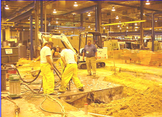
Crew drilling with wet drills for dust control.
