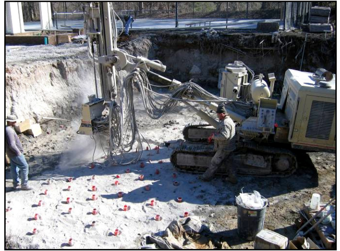
Drilling 2.5" holes with a track drill
