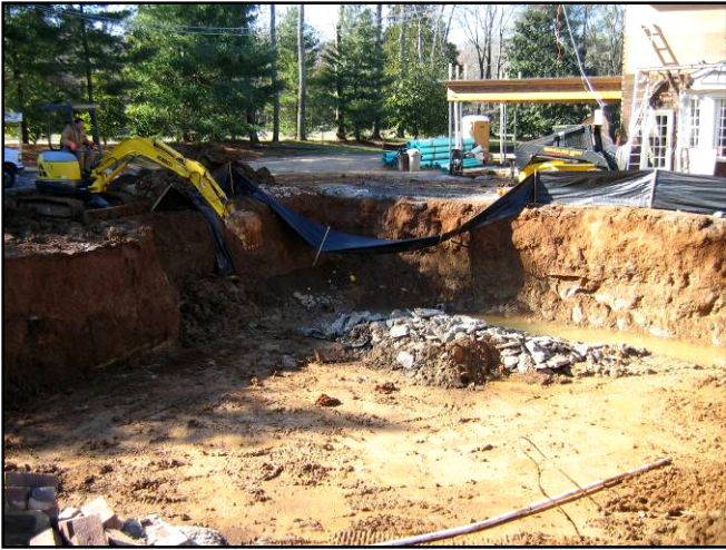
Area to be excavated. 42ft x55ft x5ft solid limestone
