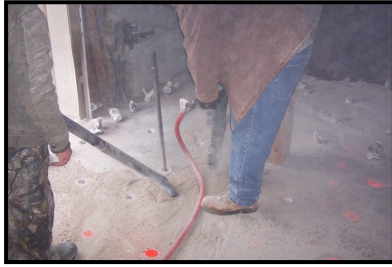
Above: Drilling 1 3/4" holes
