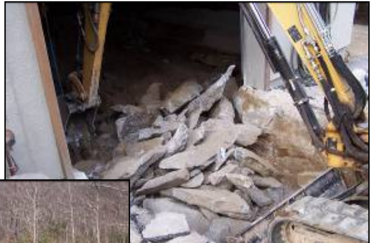
Above: Mini-excavator removing rock.
