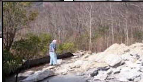
Left: Pile of Rock from excavation
